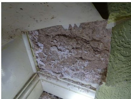
View of cracked, crumbling, and damaged plasterwork to the first floor bedroom.
