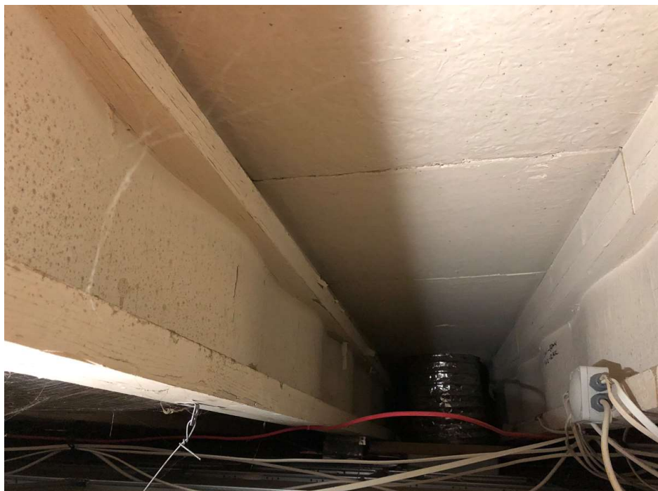
Photo 46: Woodwool roof slabs, painted white, bearing onto long-spanning engineered timber joists. This is above the former squash courts.
