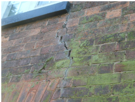
View of stepped cracking above the front elevation ground floor window.
