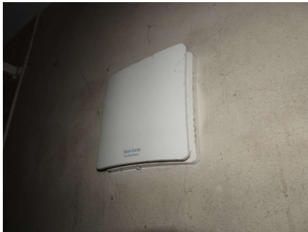
View of extraction fan to the first floor bathroom.
