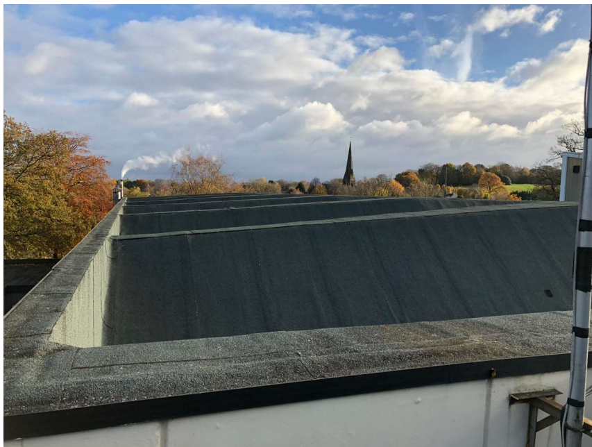
Photo 42: Roof over Main Pool. Structure projecting above. Felt looks in reasonable condition to this part of the building.
