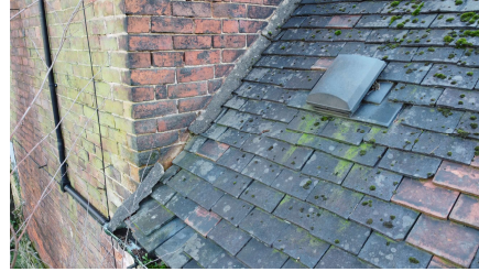
View of cracked and part missing mortar to the flashing abutment.
