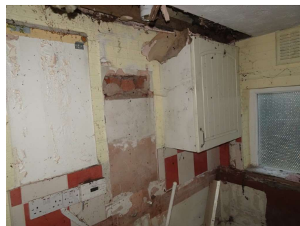
View of the damaged plasterwork to the kitchen area.
