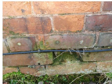
View of chemical damp proof course to the low level masonry brickwork.
