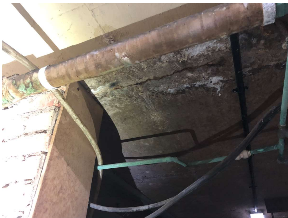
Photo 32: Example of corrosion to underside of floor slab around the swimming pool.
