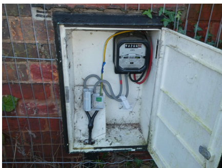
View of the incoming electricity supply and meter.
