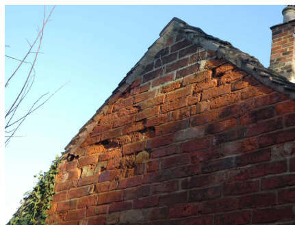
View of spalled and cracked brickwork and degraded mortar pointing.
