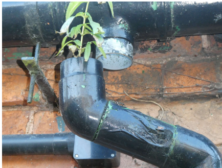
View of the disconnected downpipe to the kitchen roof.
