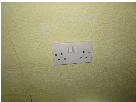
View of dated socket face plate to the first floor areas.
