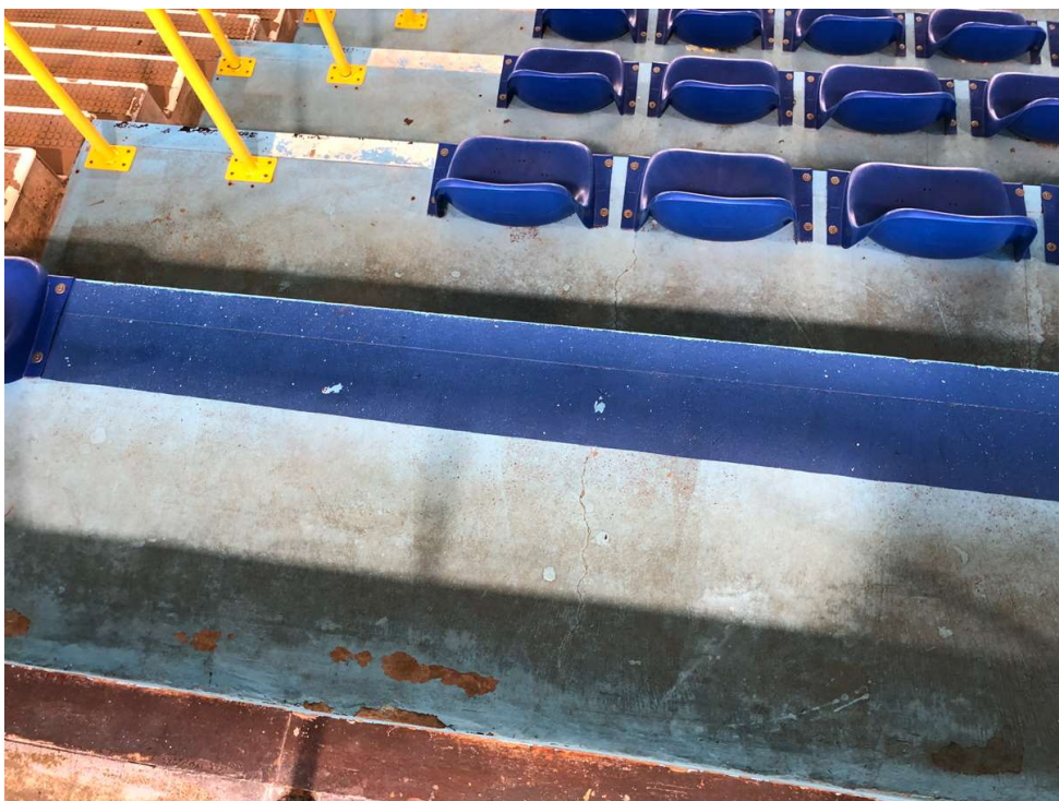
Photo 34: Hairline cracks are visible in the top and to the underside of the concrete tiered seating at mid-span. This is typical to every bay between supporting columns but is not considered structurally significant.
