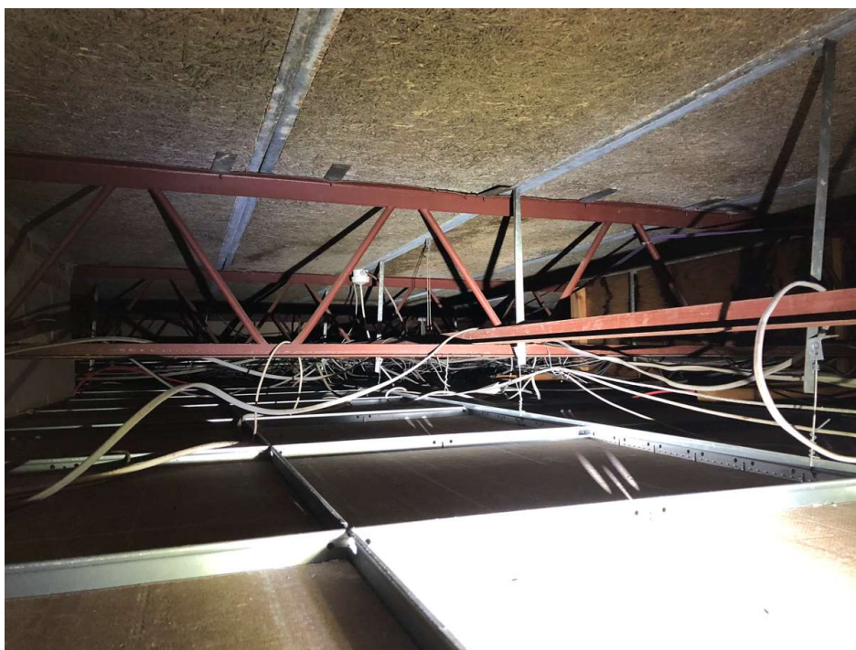
Photo 47: Woodwool roof slabs, bearing onto long-spanning steel lattice trusses. This is above the single storey fitness suite.
