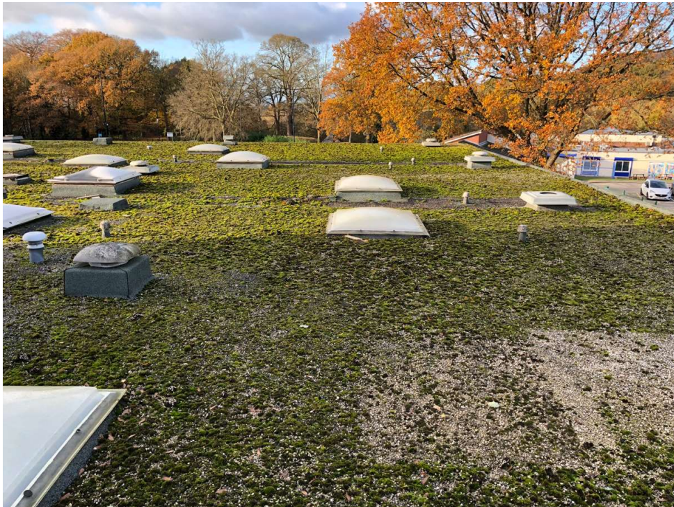
Photo 39: Flat roof over main entrance and Spa area. Heavily vegetated. The felt is in poor condition.
