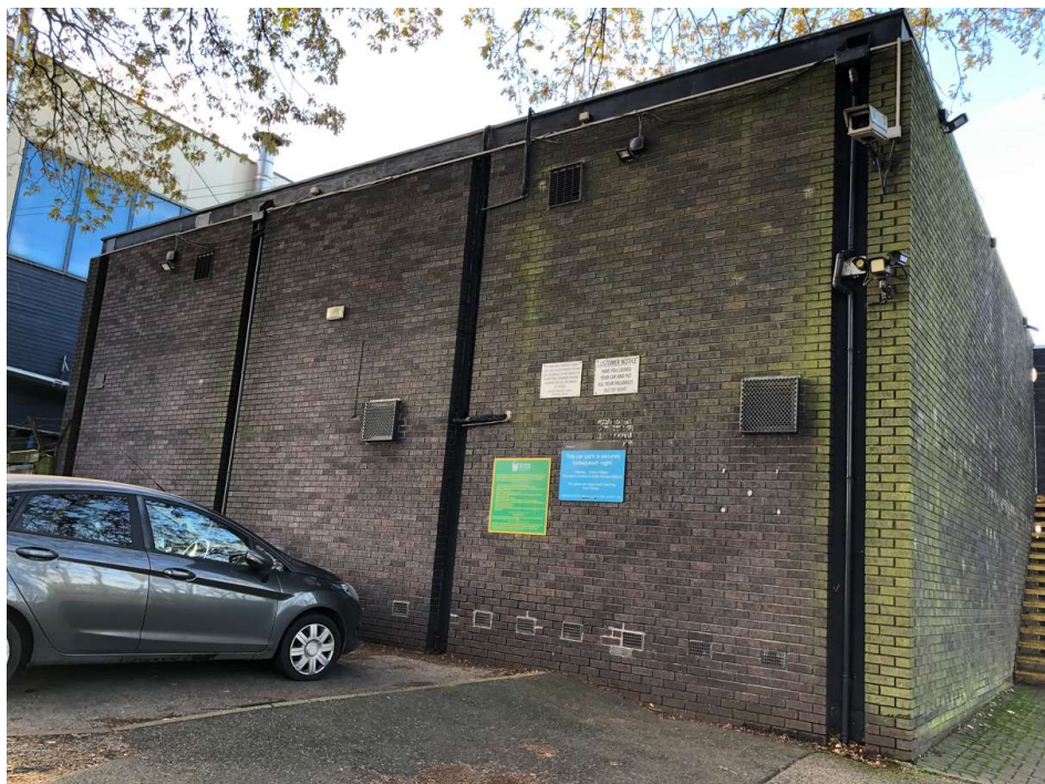
Photo 48: South (end) elevation of RAAC building. Brickwork is in good condition. The roof drains to this end and the RWPs are in recesses within the brickwork. Behind the RWPs are RAAC wall panels painted black. The roof has a small parapet.
