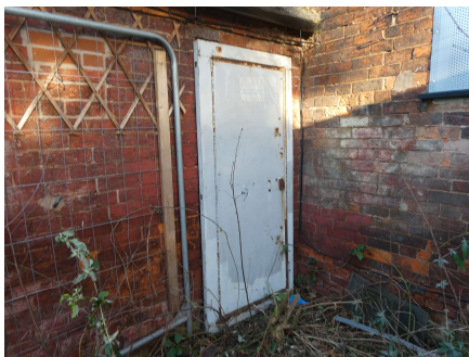
View of the metal security door installed to the brickwork in front of the kitchen door.
