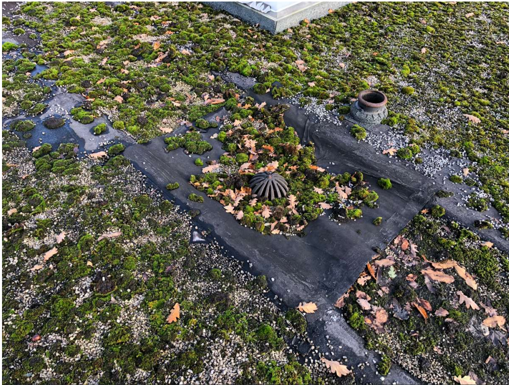
Photo 41: Failing roof felt and drainage.
