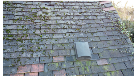
View of numerous cracked, slipped, and part missing roof tiles to the kitchen roof.
