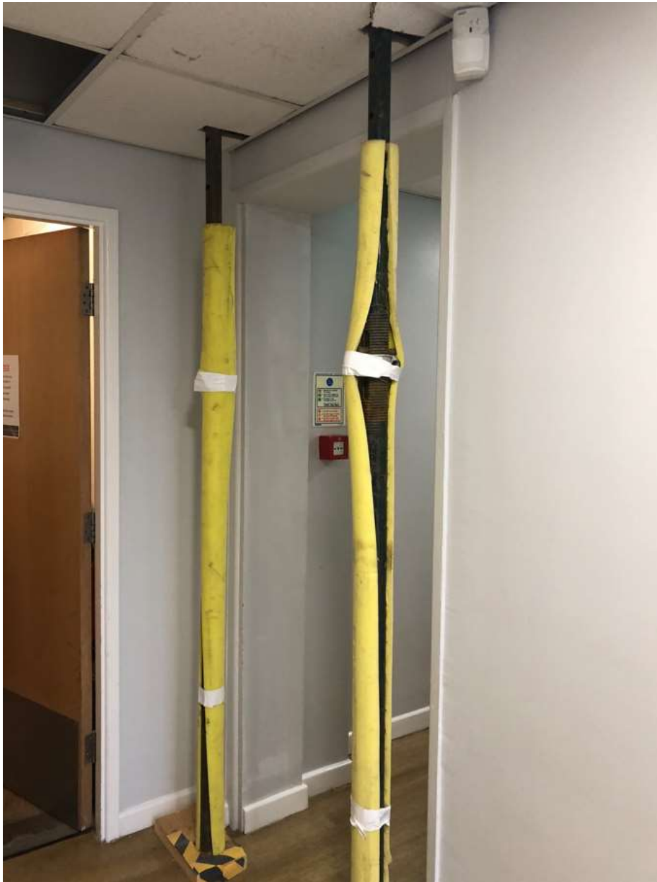
Photo 55: Since our original survey the RAAC panel has been temporarily propped as a short term 'make safe' precaution.
