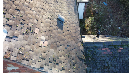
Further view of slipped and part missing slate roof tiles to the main building.
