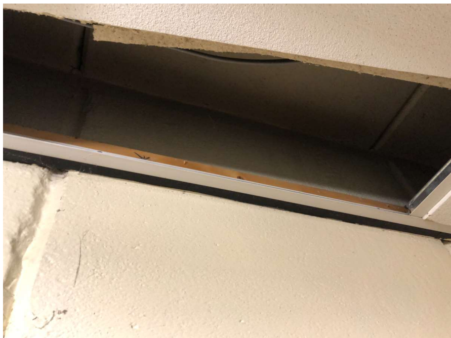
Photo 52: RAAC roof panels bearing onto RAAC wall panels. Photo taken within storeroom at first floor.
