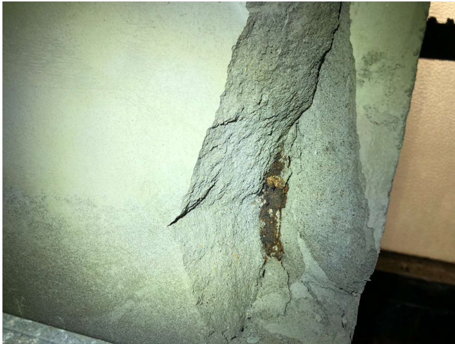
Photo 25: Corroding, expanding, steel reinforcement within the column causing the repair to fail.
