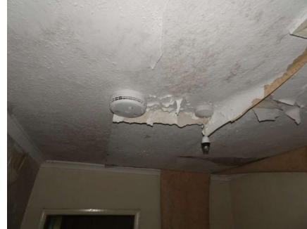
View of delaminated decorative ceiling covering to the landing area.
