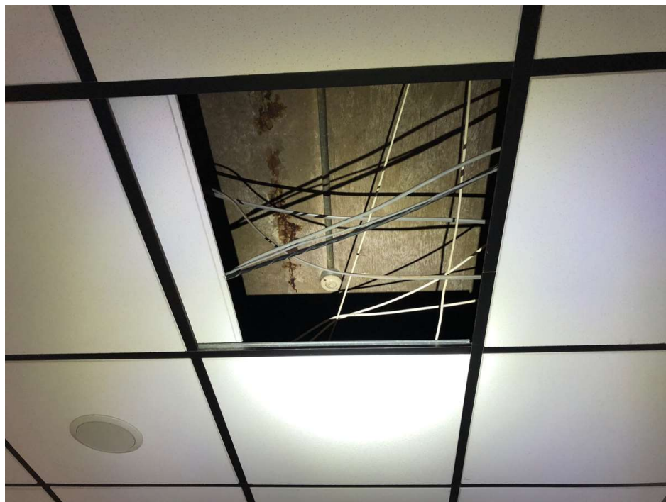
Photo 35: Underside of concrete roof slab, first floor corridor outside the changing rooms. Staining indicates corroding reinforcement due to leaking flat roof finishes above.
