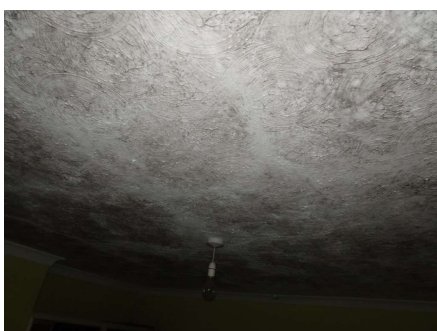
View of the mould growth and bowed ceiling to the first floor bedroom..
