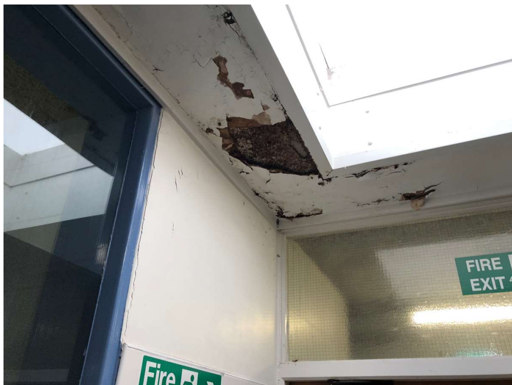
Photo 20: Staining to corridor ceiling due to a leak adjacent to roof light.
