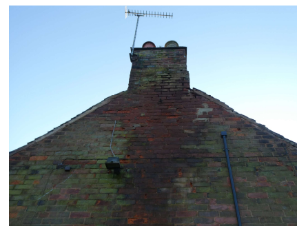
Further view of damp staining to the right hand side elevation brickwork at high level.
