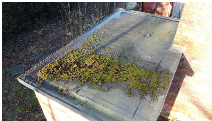
View of mineral felt roof covering to the outbuilding.
