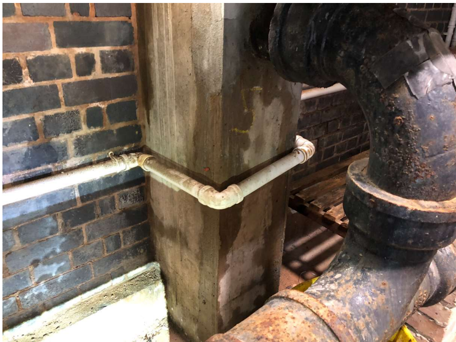
Photo 22: Typical concrete column on the southwest elevation. This column has been previously repaired but is still visibly damp. A drainage pipe, probably a roof RWP, is cast into the column. If this pipe is leaking, which appears to be the case, water will be penetrating deep into the column causing corrosion of the reinforcement.
