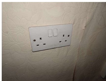
View of dated socket face plate to the ground floor areas.
