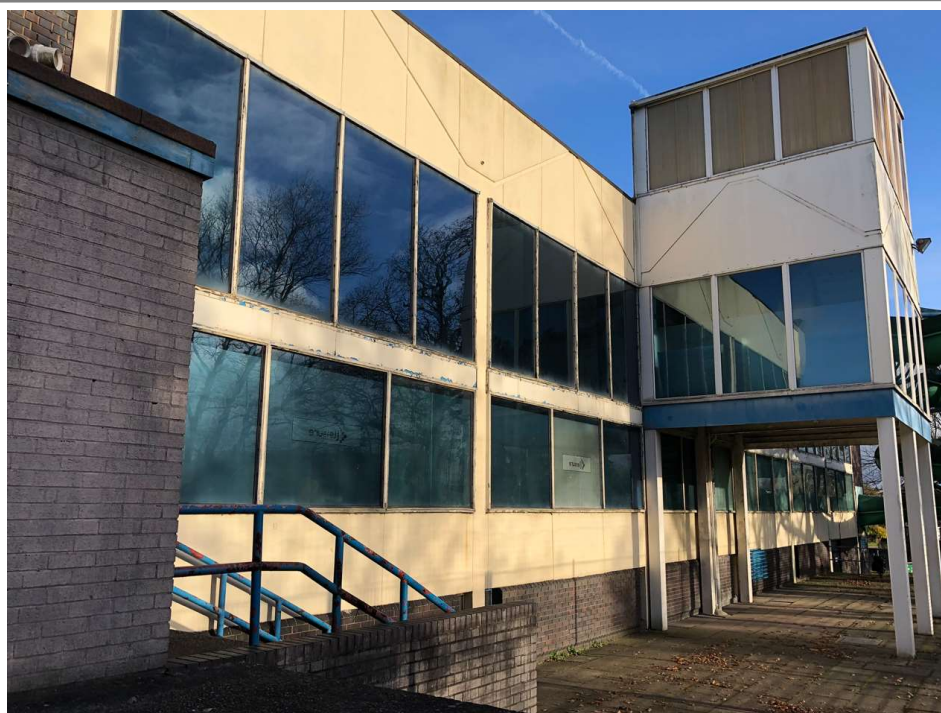
Photo 5: Southwest elevation, Main Pool. The timber framed windows are rotten and require repair or replacement. The two storey frame to the right of the photo is the access to the water slide that is no longer in use.
