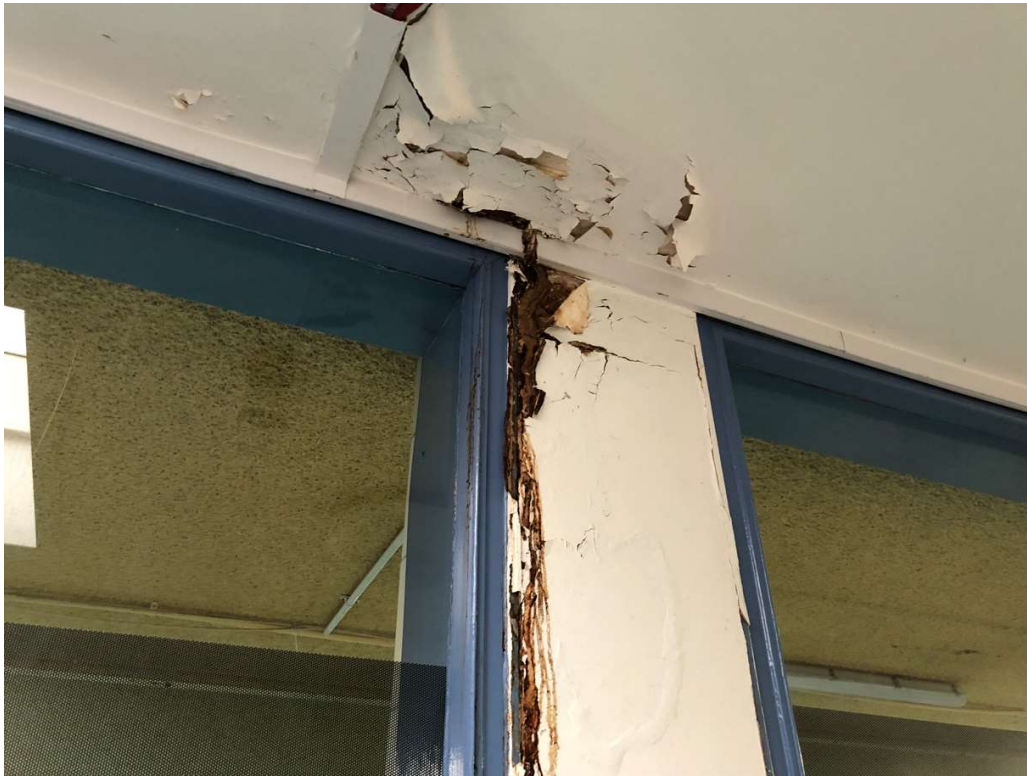
Photo 19: Roof leak causing damage at the top of an internal Teaching Pool column.
