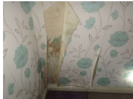
View of peeling and bubbled decorative wallpaper covering.
