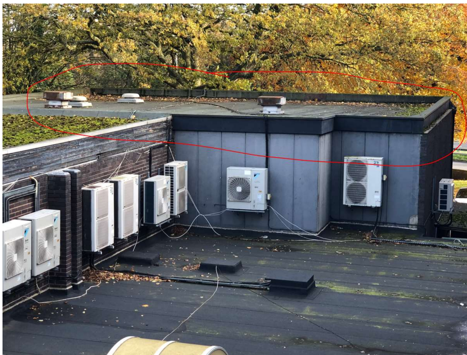
Photo 50: Roof of RAAC building. Laid to a fall towards the far end. The felt appears to be in reasonable condition. The grey vertical wall panels are RAAC.
