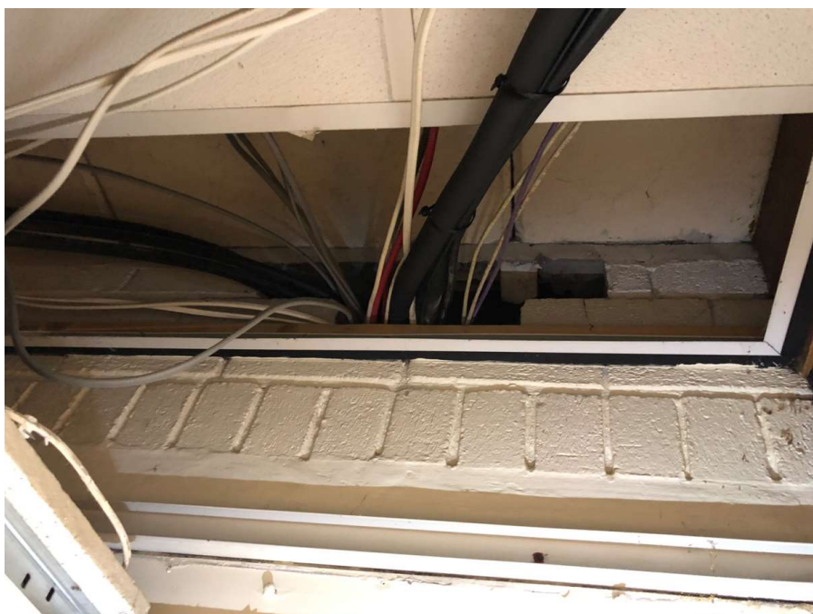
Photo 53: Lack of support to RAAC roof panel above corridor caused when service penetrations were made through the brickwork wall at high level. Urgent remedial is work required to reinstate adequate support and prevent failure of the panel.
