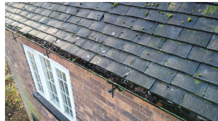
View of the PVCu rainwater goods to the front elevation.
