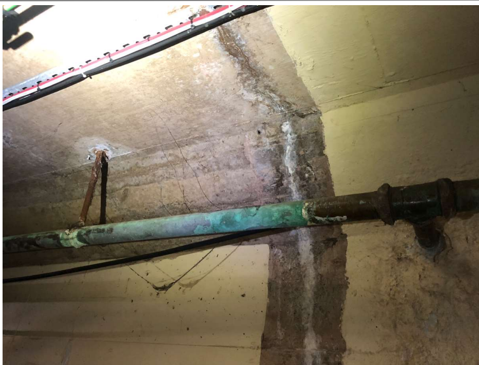
Photo 31: Main Swimming Pool tank. Vertical cracks are present in the walls. These are not considered structurally significant but should be surveyed annually to check their severity does not change.
