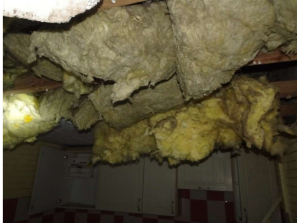
View of the collapsed kitchen ceiling.
