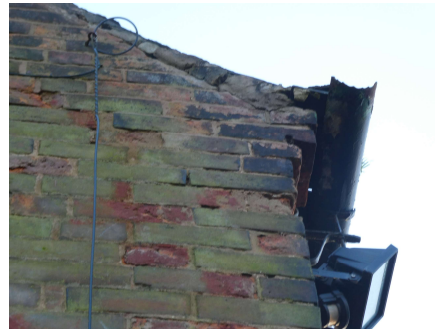
View of corroded and part missing cast iron gutter.
