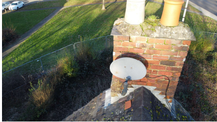
View of cracked and heavily soiled mortar flaunching to the chimney stack.
