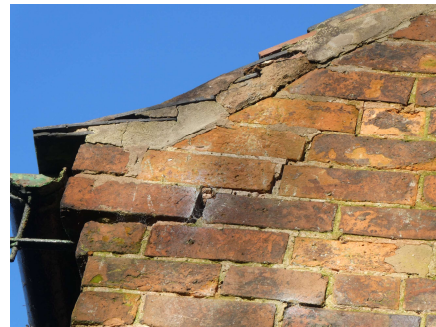
View of the cracked and distorted brickwork to the high level gable end.
