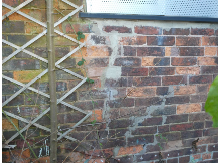
View of the cracking to the rear elevation external brickwork at low level.
